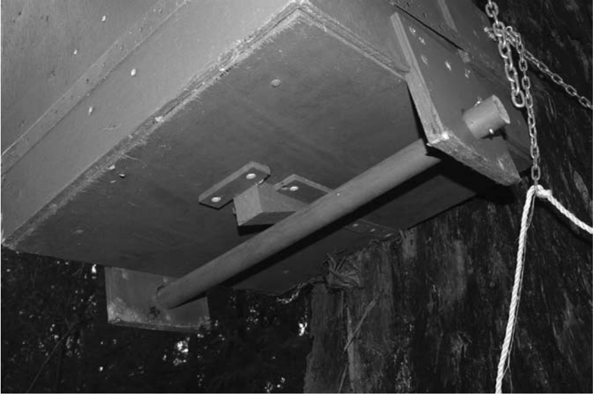
A wooden wedge is used to secure the base and create a domed floor to facilitate drainage
